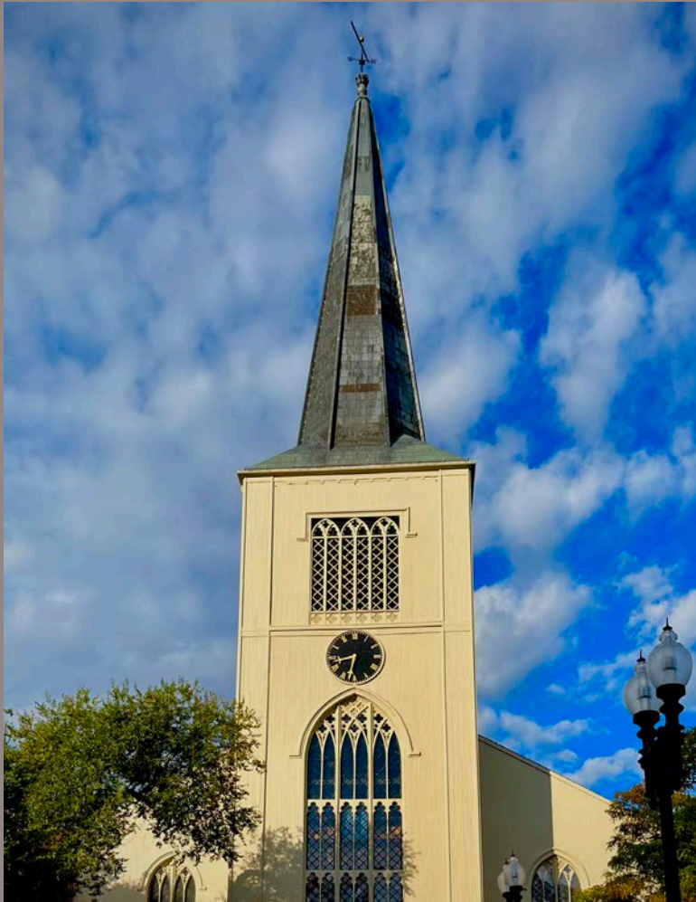
First Parish in Cambridge - 1833 Restoration Phase I - 2023
